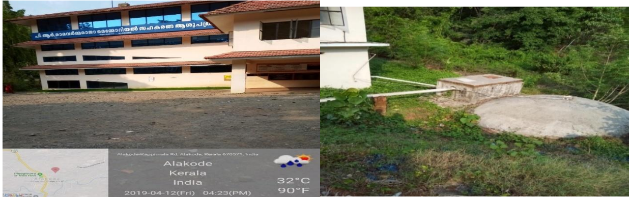
Hospital on the bank of the river (Alakkodu GP)
