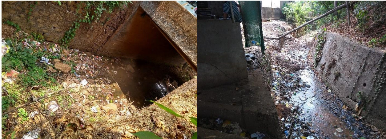
Drain of Chapparappadavu River
