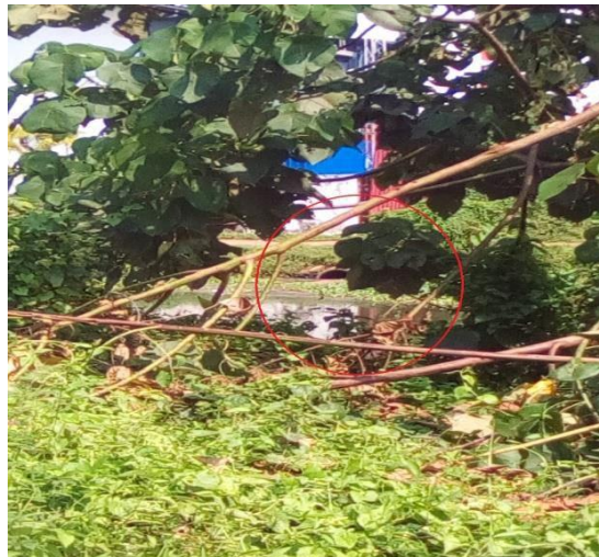
PIPE CONNECTED TO EDACHIRA THODU FROM THE NEARBY FLATS
