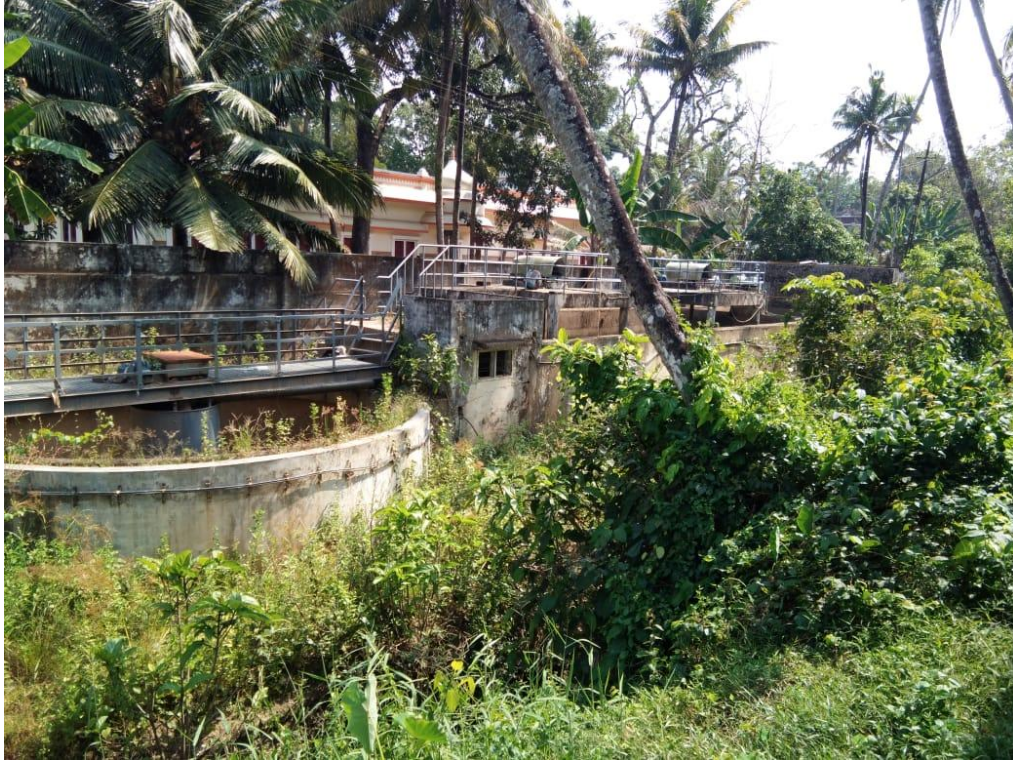
Non- Operational STP of Aluva Municipality near Ashramam
