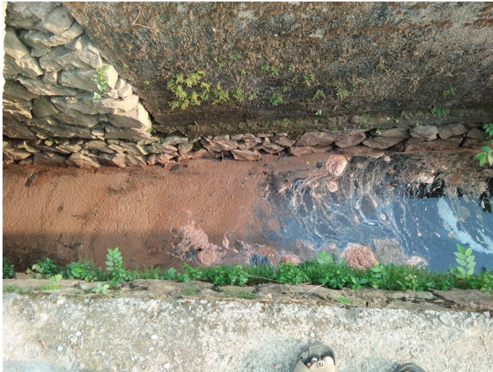
Drain carrying Sewage from Kalamassery Market joins at Periyar river at Puthalamkadavu
