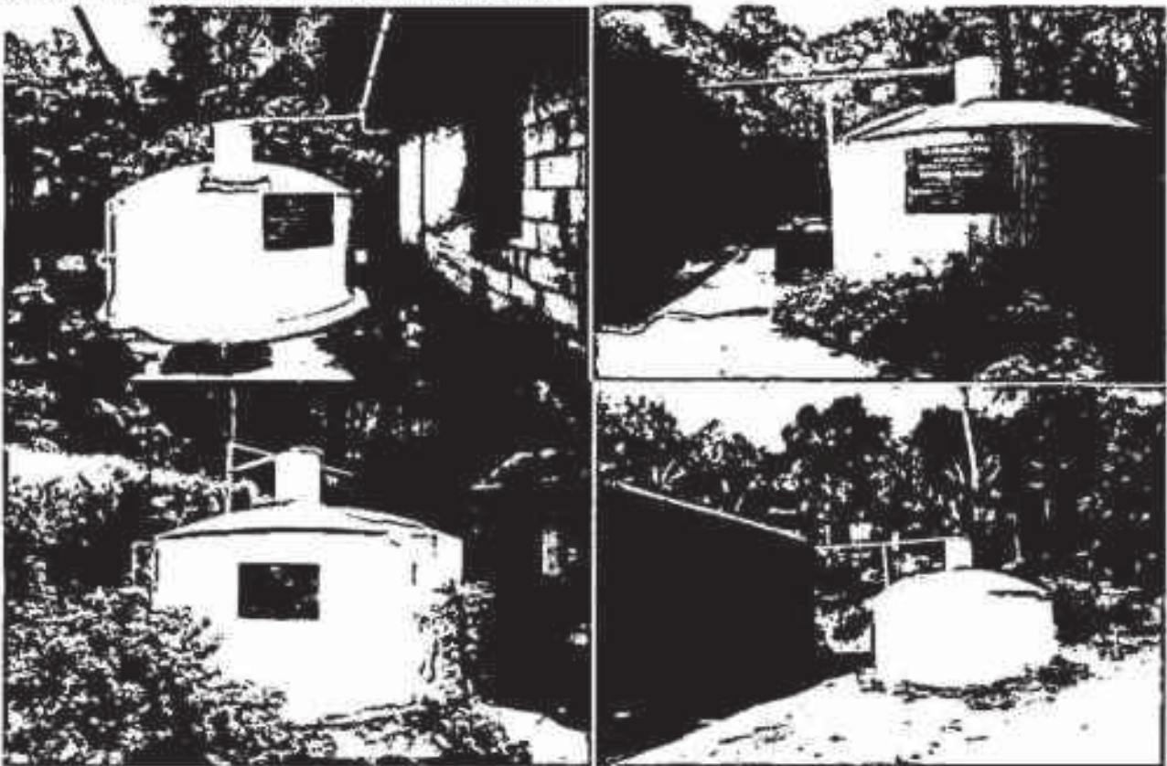
RWH units constructed in individual households.
