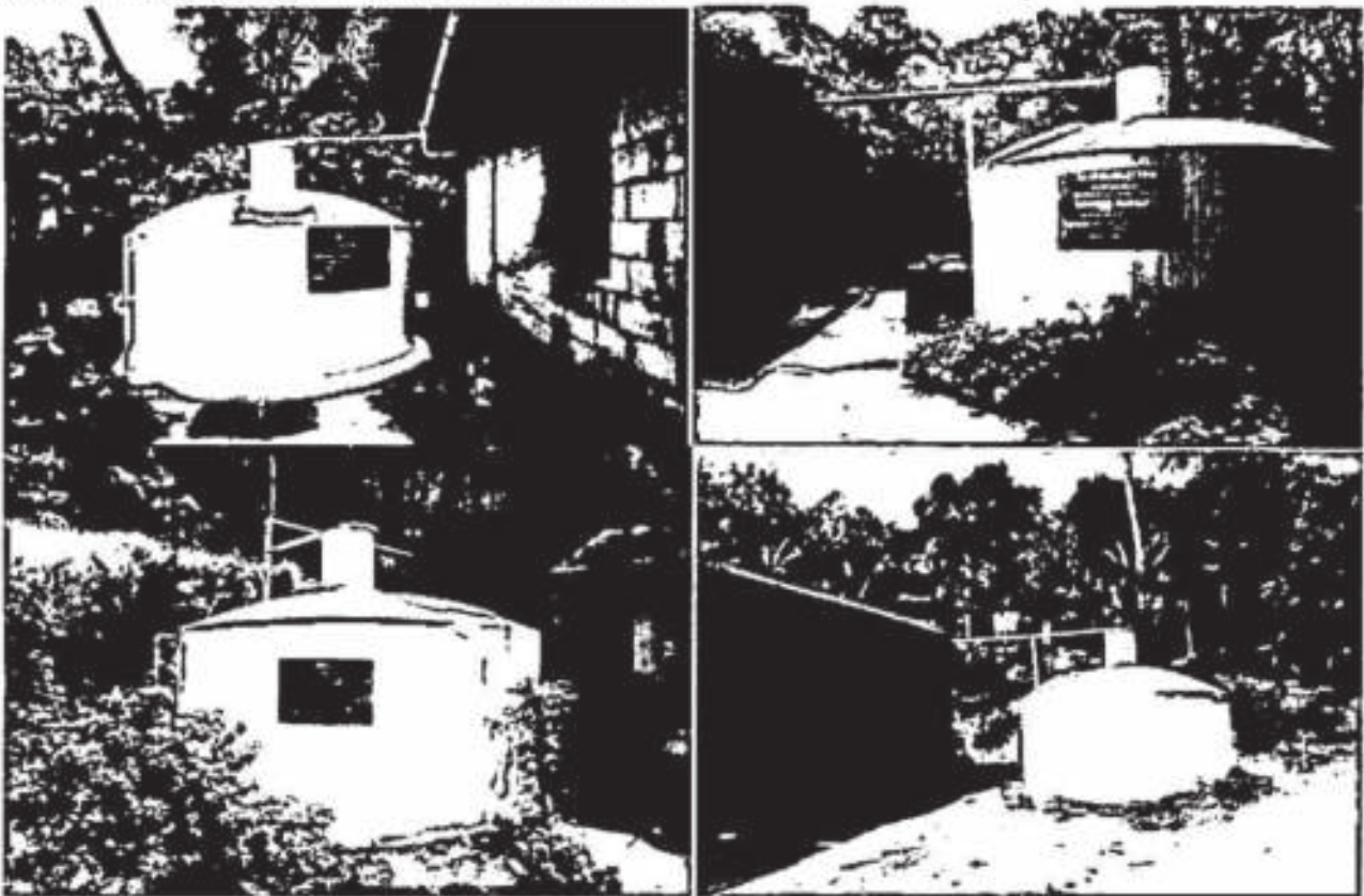
RWH units constructed in individual households.
