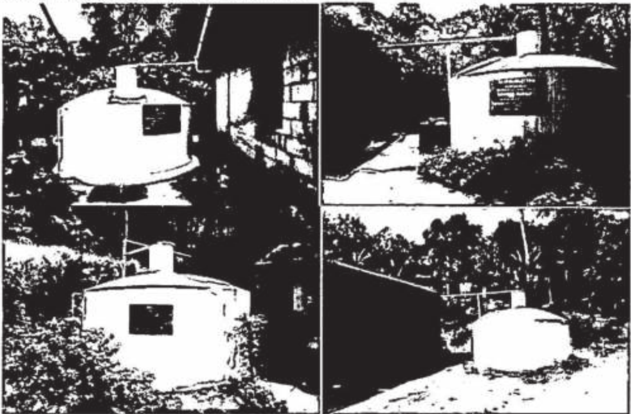
RWH units constructed in individual households.
